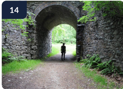
As you approach the car park, head towards the tunnel which runs underneath the railway line.
