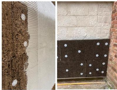
33 Application of Cork Board and render coats.
