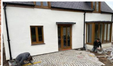
35 Following application of lime render and breathable paint.
